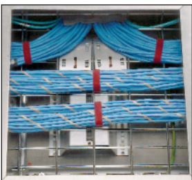
Underfloor (Plenum application) HLSP3S-X12 HLTP3I-X12
