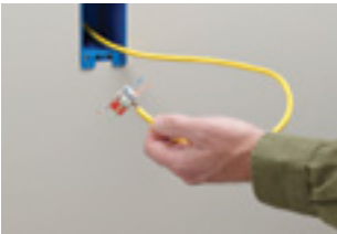
2. Determine wiring scheme. Dress all four pairs (eight wires).
