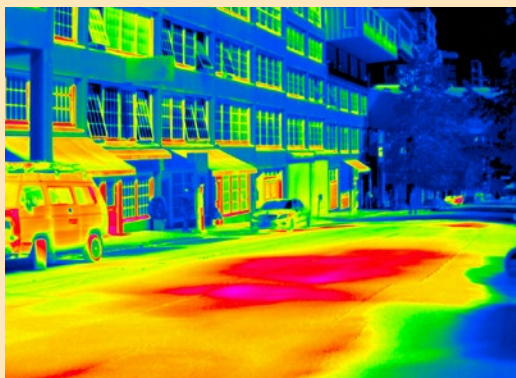
Steam vents under city street
